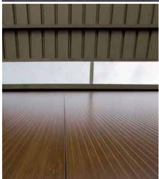
Detail of the internal side
