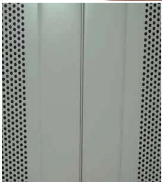
Detail of the roof
