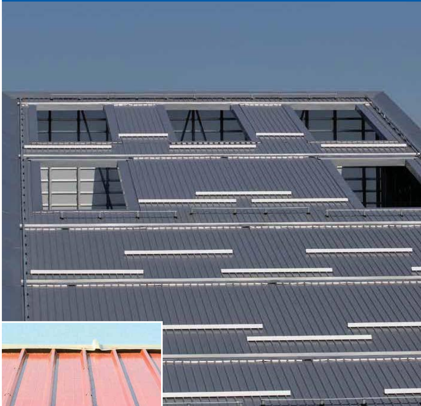
Roof of a management centre in Milano
