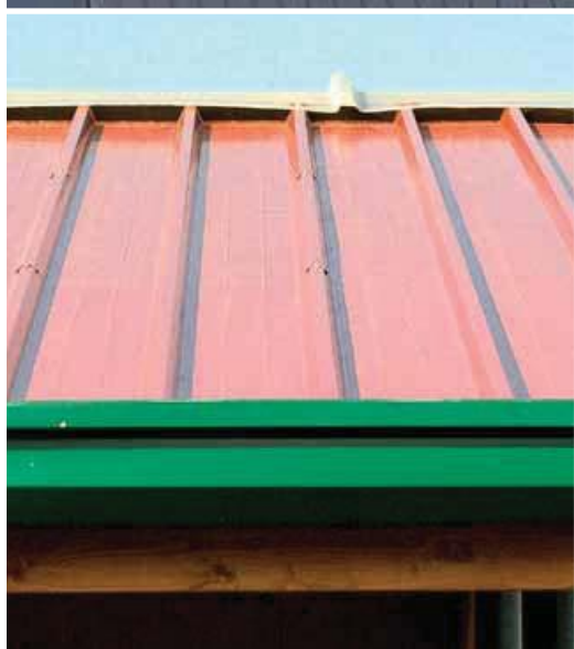
Detail of the roof
