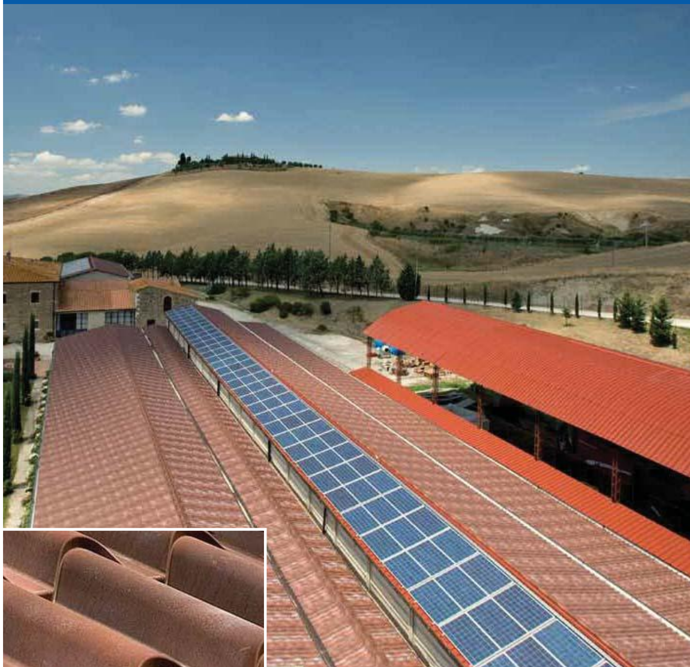
Renovation of an agricultural building in Pienza
