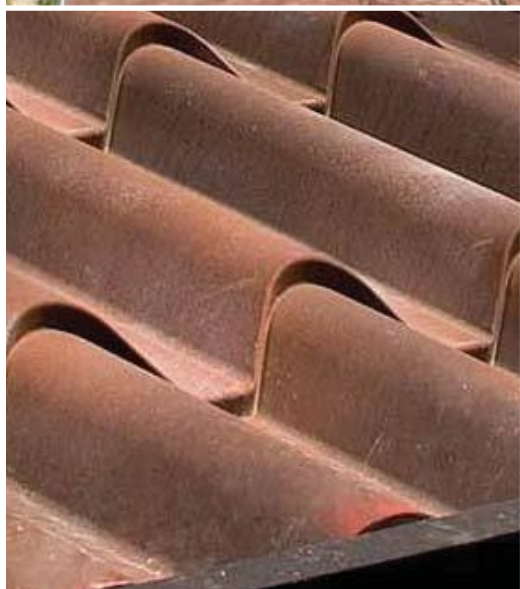
Detail of the roof
